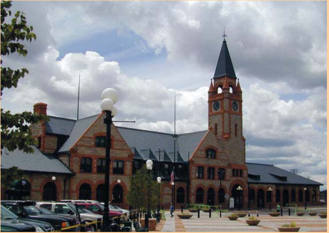
Public facilities can also serve as landmarks, as they are often have distinctive architecture and are located on prominent sites.
